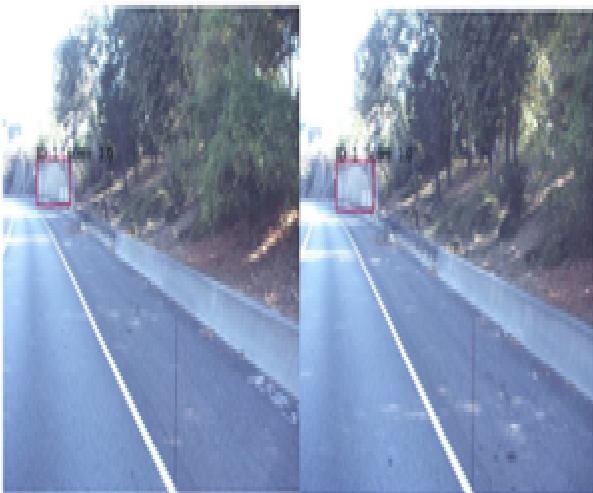
Figure 4: Tracking to Cluster the Same Retaining Walls at Different Roadway Images
